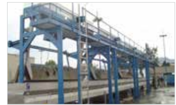
Cable Operated Bar screen
